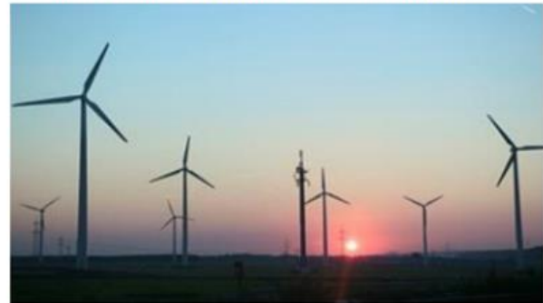
26 MW Wind Power Project at Jaisalmer, Rajasthan
