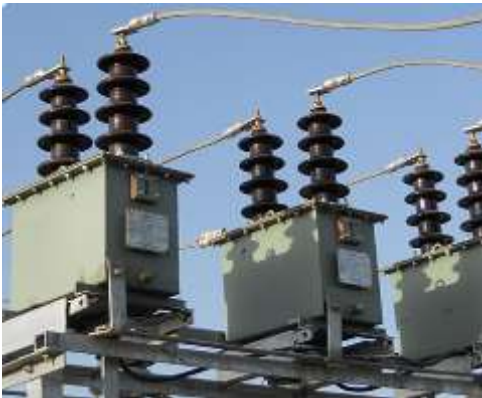
MV Current and Voltage Transformer upto 33 kV
