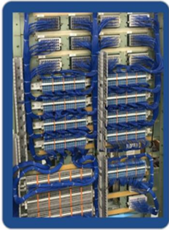
Railway Signalling Panel
